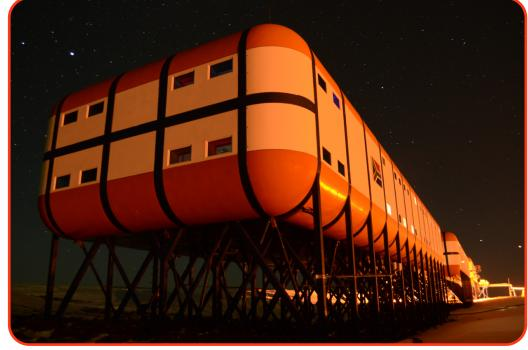
further stayed with 4 or 5 anchors to keep them in place. The framework was then welded onto these sunken foundations.
